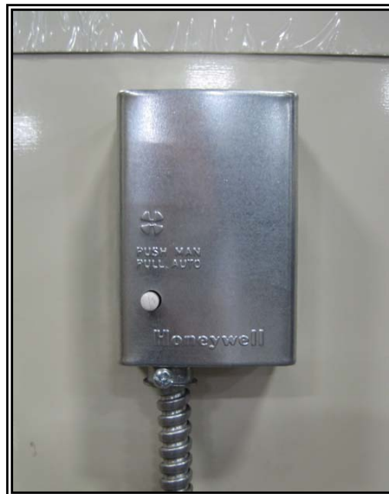
Figure 9: Fan/Limit Control, Mounted
