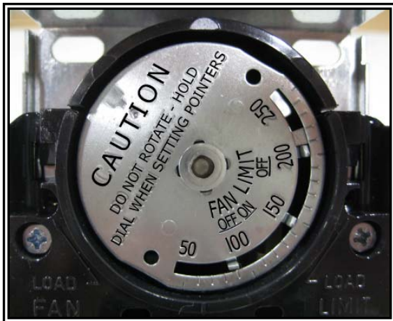
Figure 10: Fan/limit Control Settings Recommended “Fan Off” setting is 90 ° F. Recommended “Fan On” setting is 145° F.
